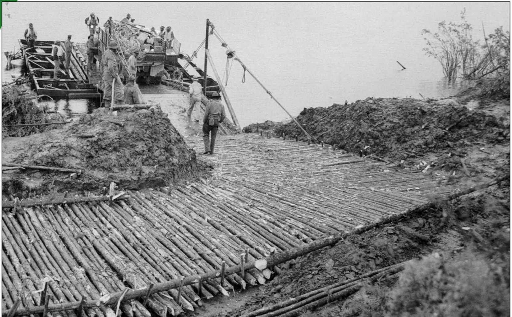
Corduroy road surface under construction.
