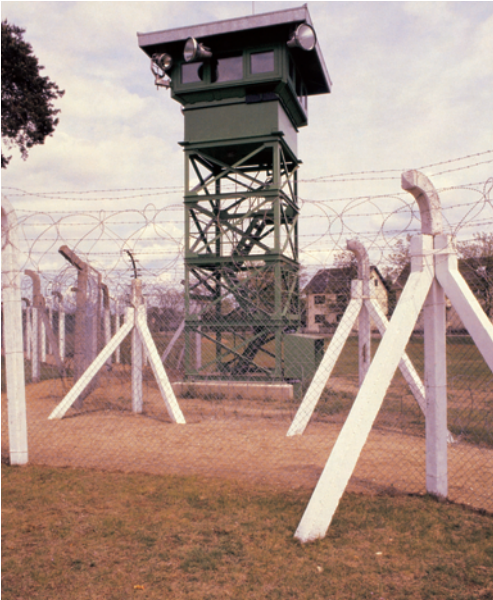
The Europe Division generally relied on contractors to complete facilities, such as this prison in Mannheim.
