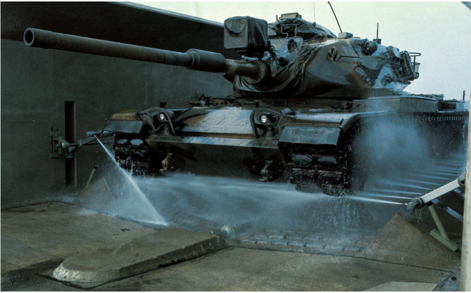
Army engineers also constructed washracks for tanks, trucks, and other vehicles.
