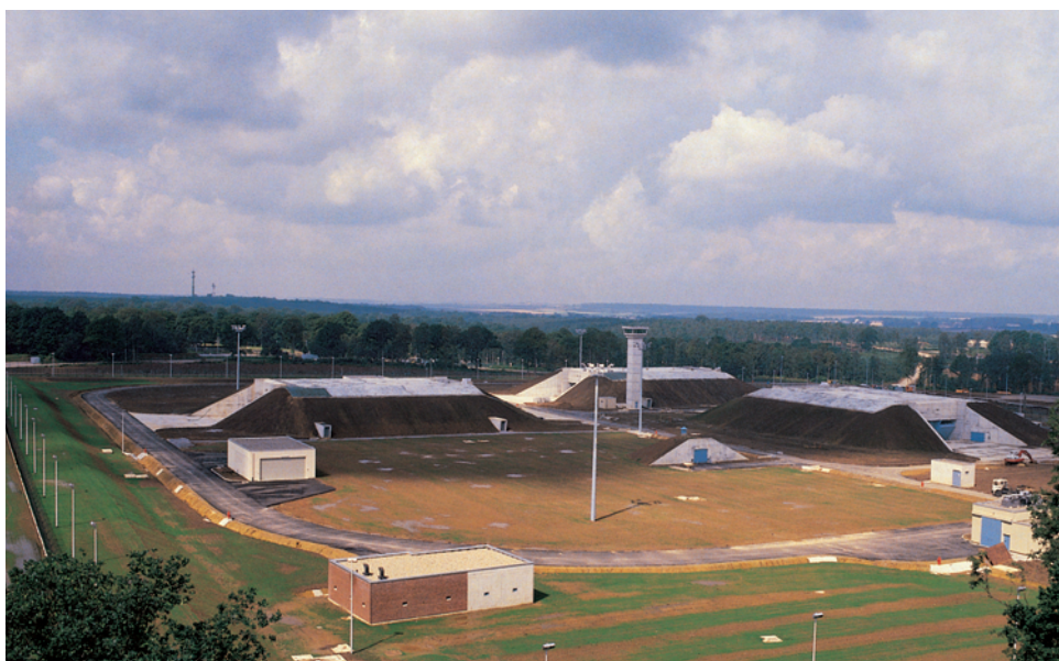
GLCM sites in Western Europe, such as Florennes, Belgium, included support and operational facilities.
