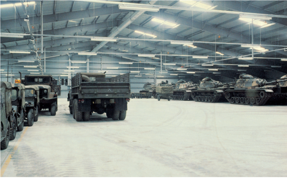
Vehicle shelters, like this one in Mönchengladbach, Germany, were an integral part of the POMCUS and POMSS construction programs.
