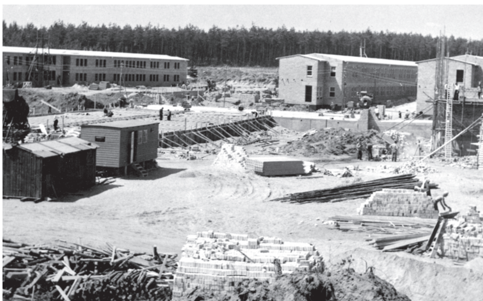
Medical Facility under Construction in Landstuhl
