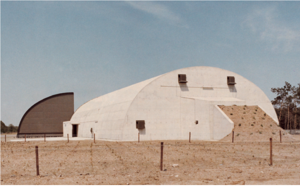
Aircraft shelters resistant to atomic attacks were constructed in 1976 and 1977 in Gilze-Rijen in the Netherlands.
