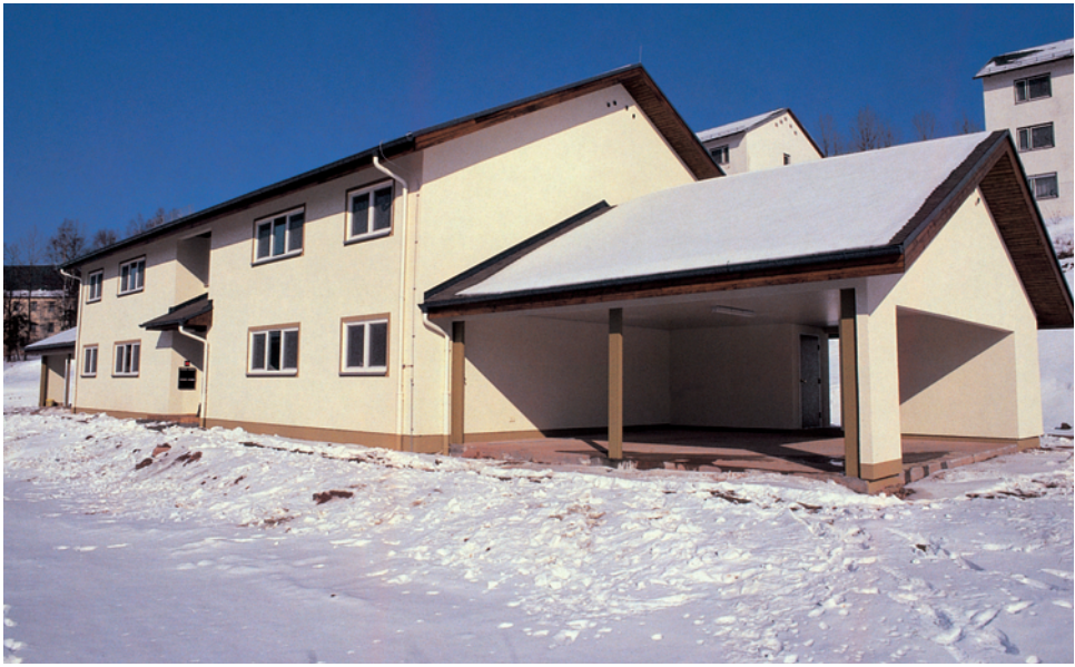
Prototype of Prefabricated Housing on Site in Wildflecken, Germany
