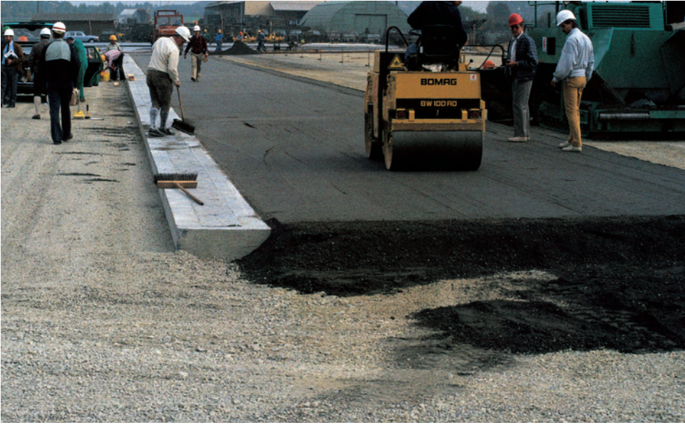
Roller-compacted concrete was used to construct hardstands in Kitzingen, Germany, in 1986 and 1987.
