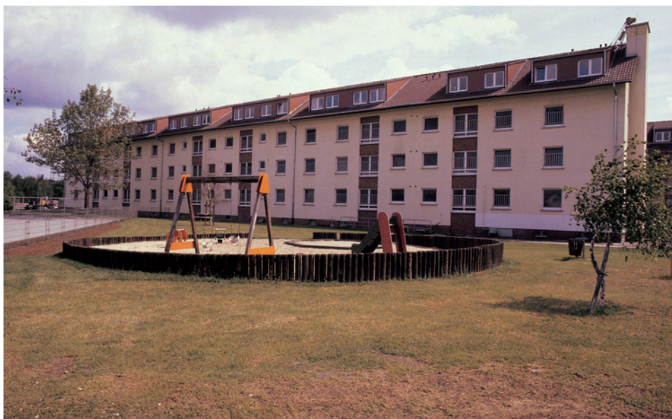
Although the roof line of this housing unit in Mannheim, Germany, was altered to add apartments in the attic space, the footprint of the building remained the same.
