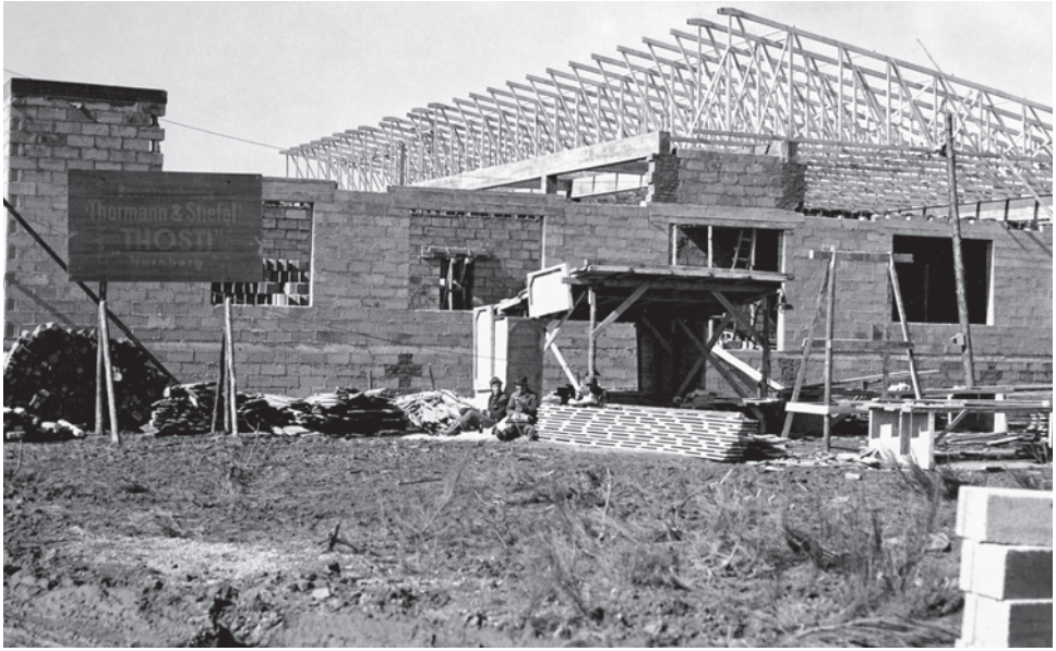
Construction of a Shipping and Receiving Warehouse near Kaiserslautern, March 1952
