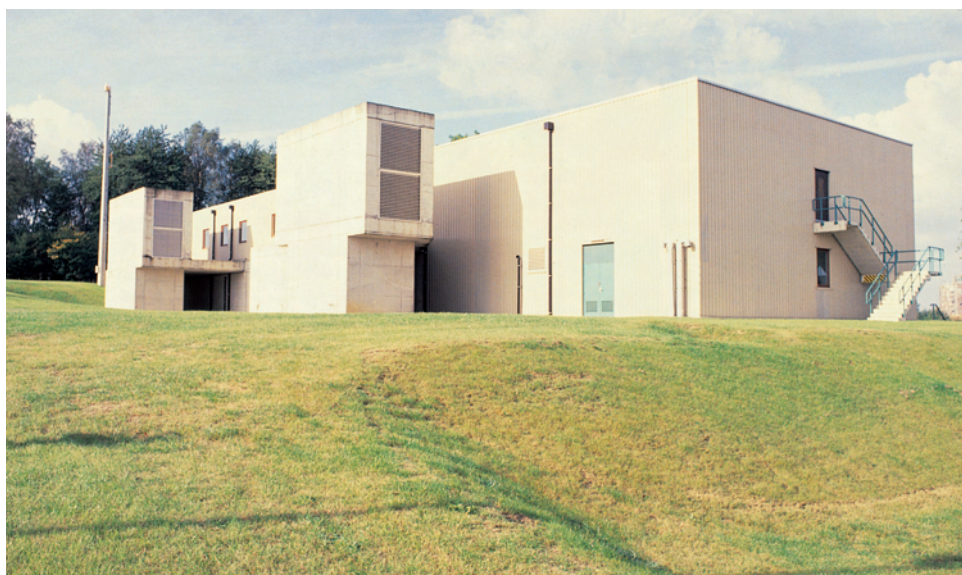
The Northern Area Office was responsible for this headquarters building at an air base in Florennes, Belgium.
