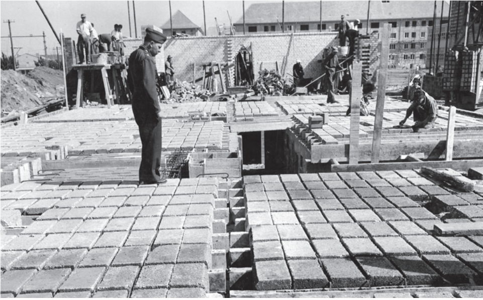
Engineers used ribbed-concrete floor construction for housing in Mannheim, Germany.
