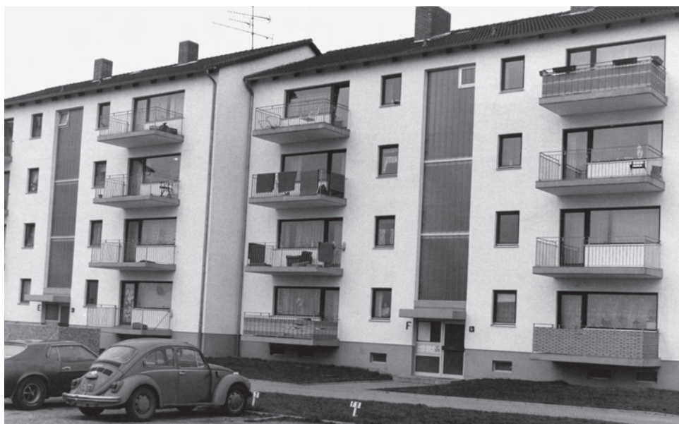
Europe Division workload included build-to-lease family housing projects for the Hanau community.
