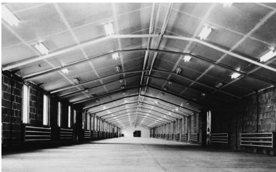
Army engineers built depots like this one in Hanau to store equipment arriving in Germany as U.S. troops moved out of France.
