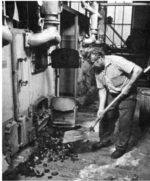
Coal-fired boilers, like this one at Warner Barracks in Bamberg, were prevalent in the 1960s and 1970s.
